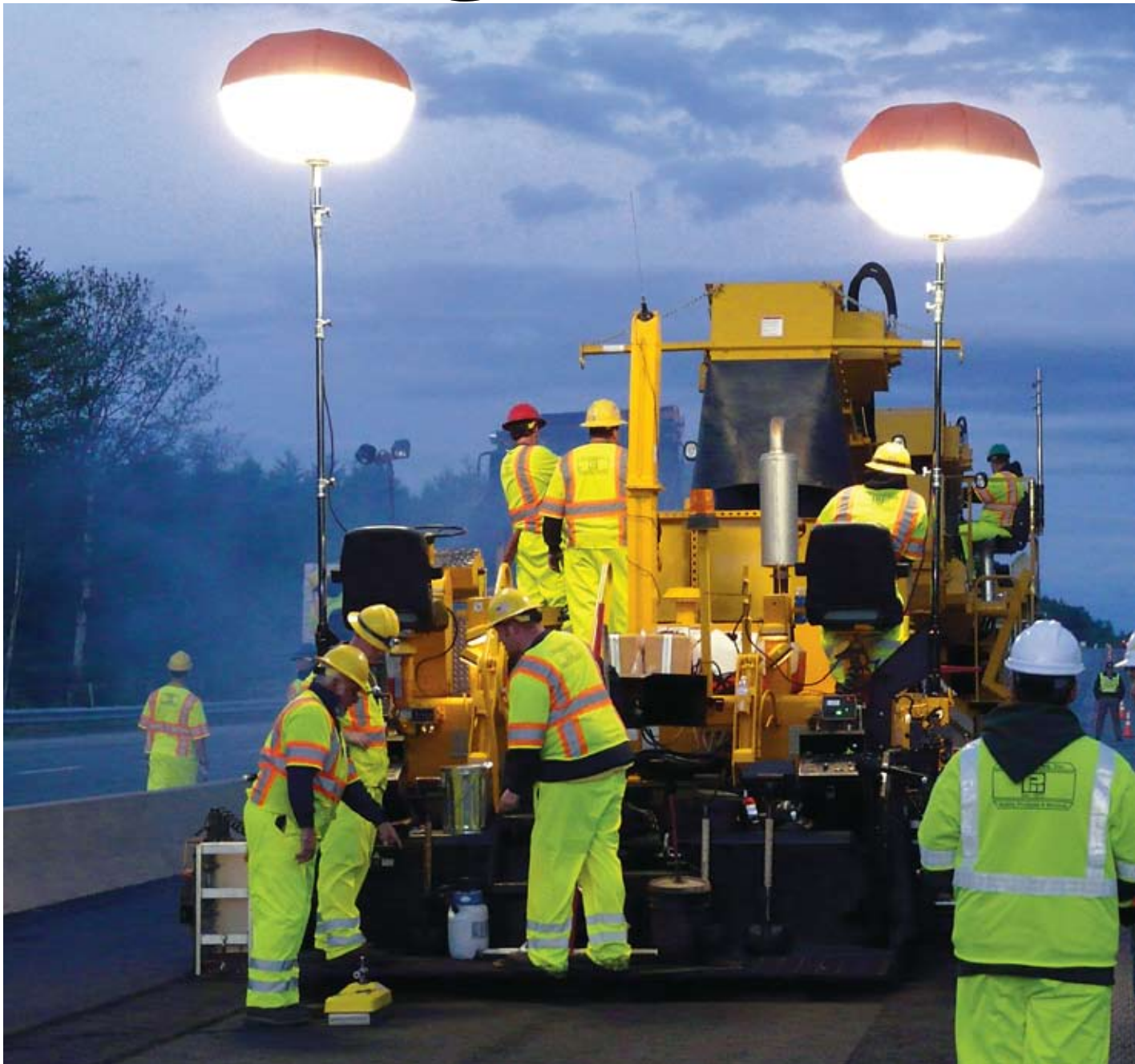
▲ Night Moves. Pike Industries Inc. paving crew working on a New Hampshire ARRA-funded highway job; the state mobilized quickly to get projects ready.
